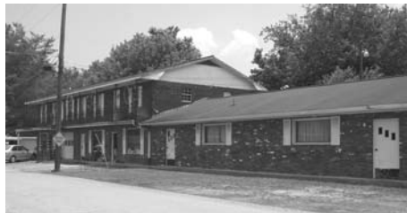
Existing Lenoir City building, recently purchased by the Domestic Violence Crisis Center.
